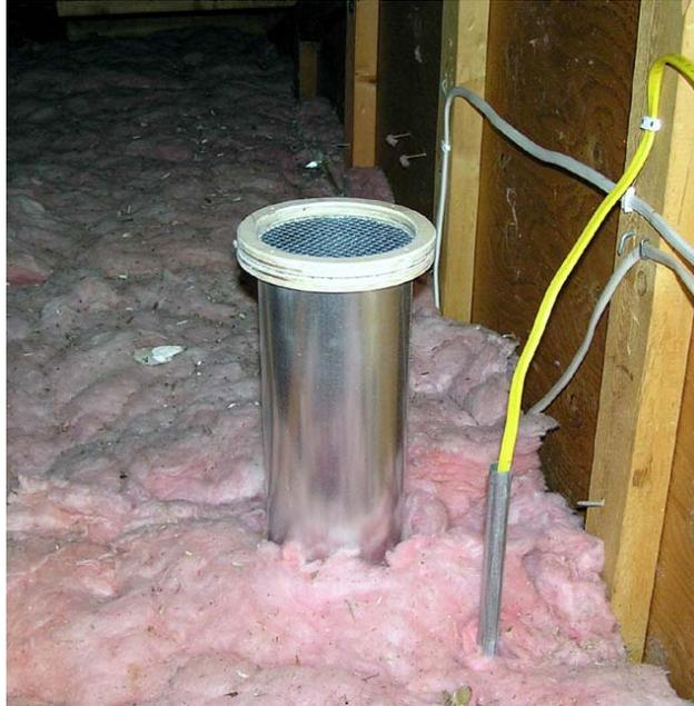
I fabricated a simple screen for the discharge pipe from two rings of birch plywood and a little  $\frac{1}{4}$ -inch mesh hardware cloth. This should keep the larger “critters” out; anything small enough to get through the mesh will be in for a bit of a surprise when the blower fires up:
