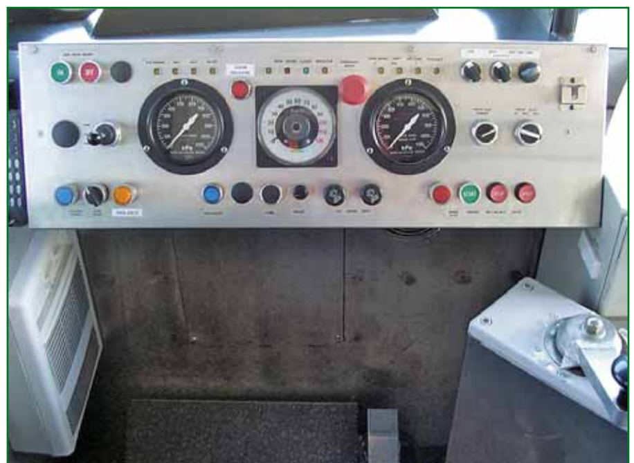
▲ The newly refurbished driver's panel.
