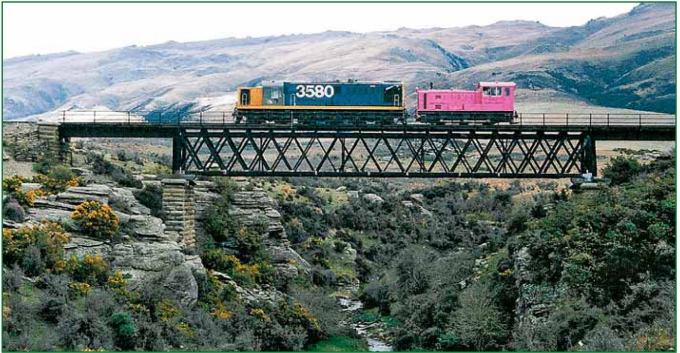
▲ The real 5 Mile Creek Viaduct in Central Otago, taken during the last few months that it still had a railway line on it. The track demolition train locos are crossing it (June 1991).
