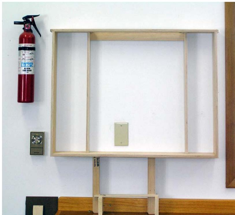
Then I glued and bradded the back on permanently.<sup>2</sup> When dry, I hung the filter cabinet with two 1/4" lag screws through the mounting ledger into wall studs:
